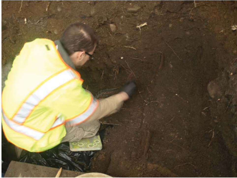
Figure 12. Excavation in progress.
