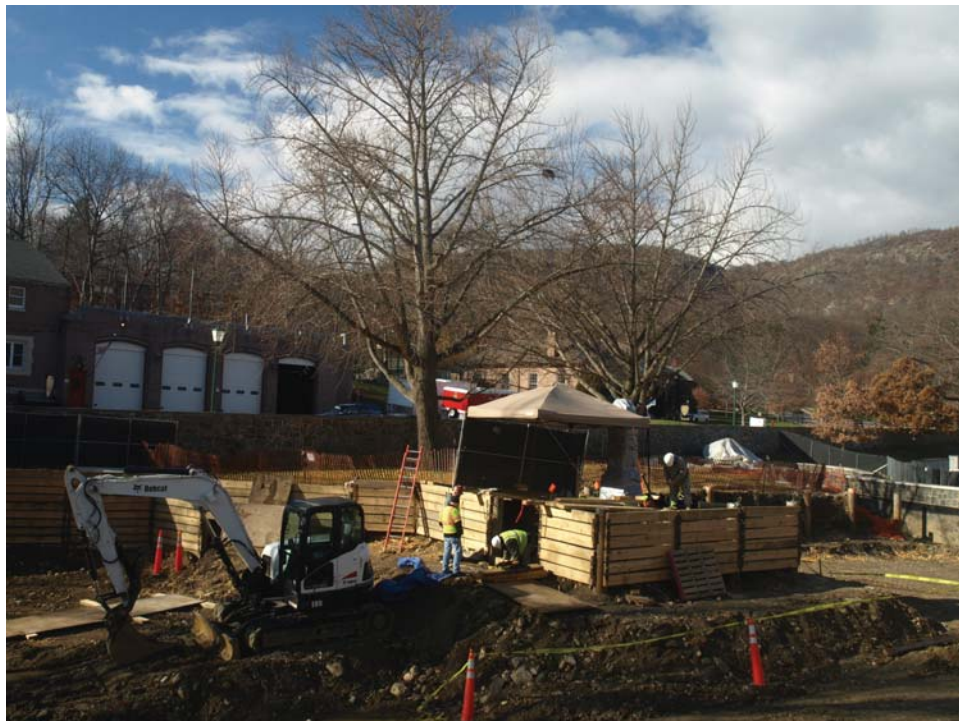
Figure 3. Overview of project area showing location of burial, facing northwest.
