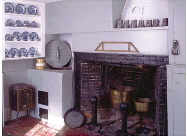
The home was built with a scullery where household staff prepared food and did laundry. The room contains a unique set-kettle (left) fitted with a drain so it could be emptied to the outside instead of indoors.
